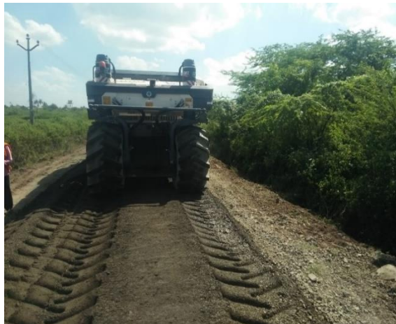
Figure 2: Recycling of base course
