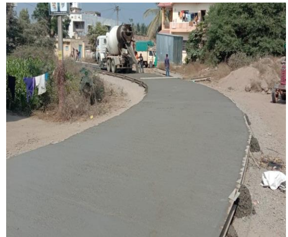
Figure 3: Laying of PQC
