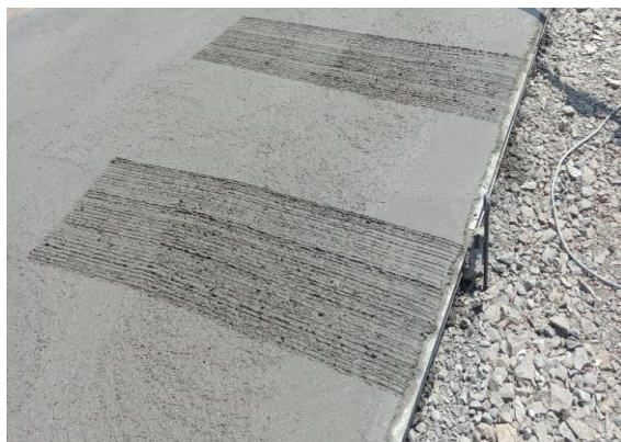
Figure 4: Texturing of Concrete
