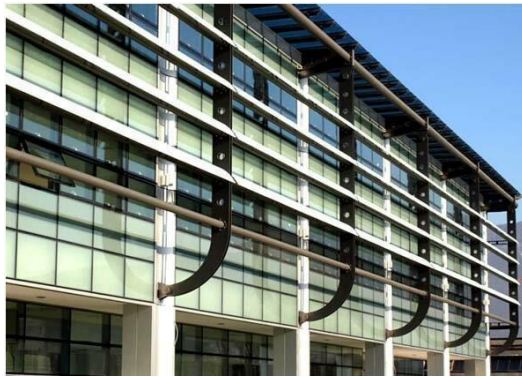
Figure 8 Brise soleil - shading devices integrated with the building façade, Source: (Maleki, 2011)
