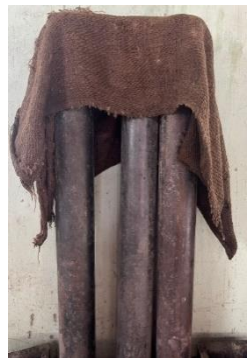
b) Curing of CFST column
