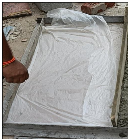
Figure 2.1 Preparation of formwork
