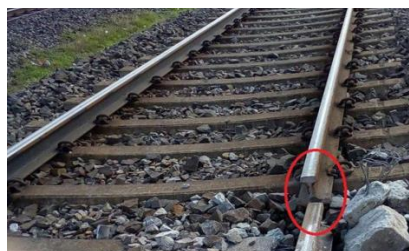
Figure 1: Crack on the railway track
