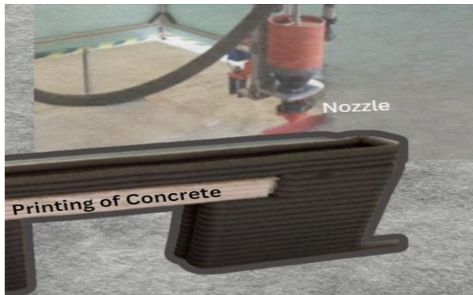
Fig 5: 3D Printed wall up to lintel.
