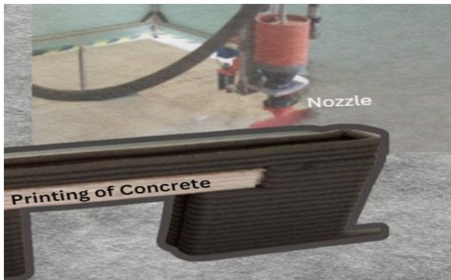
Fig 5: 3D Printed wall up to lintel.
